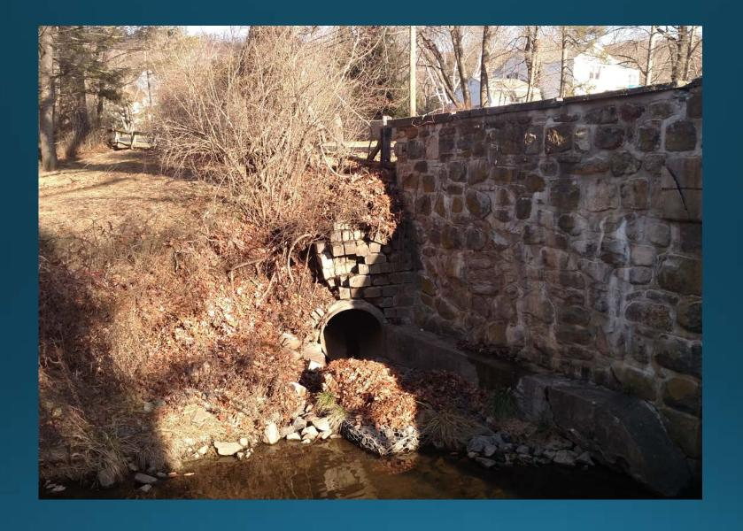
Crumbling headwall on downstream channel
